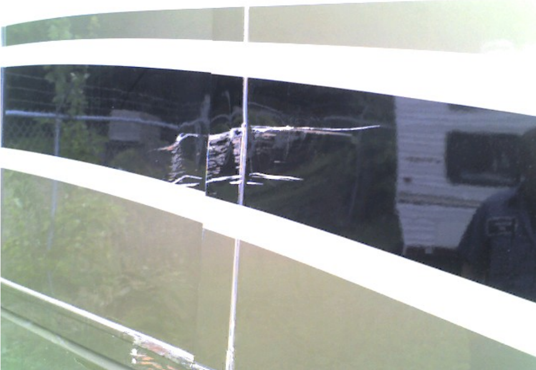
Damage to gel coat and paint (Fiberglass broken zoom in to view)
